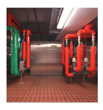
end" portion of the meat. It is also possible to add intermediate stops and to decide their duration. Suction ducts are mounted to the ceiling where air flow is controlled by micro-adjusting valves. This kind of system is designed to operate at a low relative humidity, to obtain a high dehydration of the ham at low temperature, thus preventing bacteria from developing and allowing the salt to penetrate into the heart of the raw ham.
